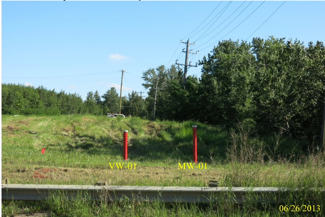
Photograph No. 7: View of completed wells MW-01 and VW-01, looking south.
