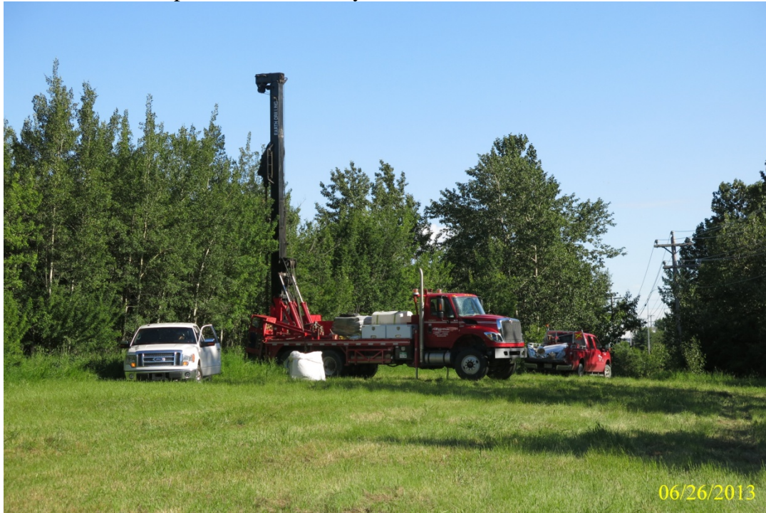
Photograph No. 9: Drilling VW-02, located at the southeast site of the site. Note truck mounted auger drill.
