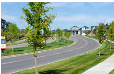
Example of separated sidewalk.
