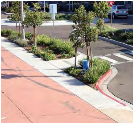
Coloured concrete in median paving area.
