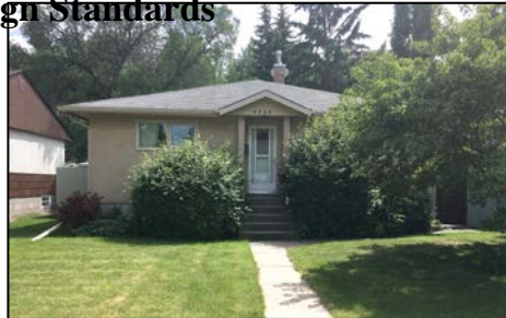
Typical Bungalow with Hipped Roof
