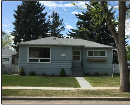
Typical Bungalow with Hipped Roof
