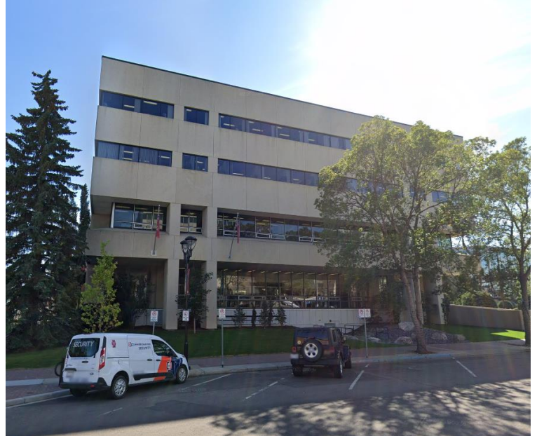
Side of building (north elevation)
