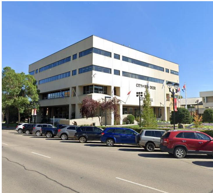
Back of building (west elevation)
