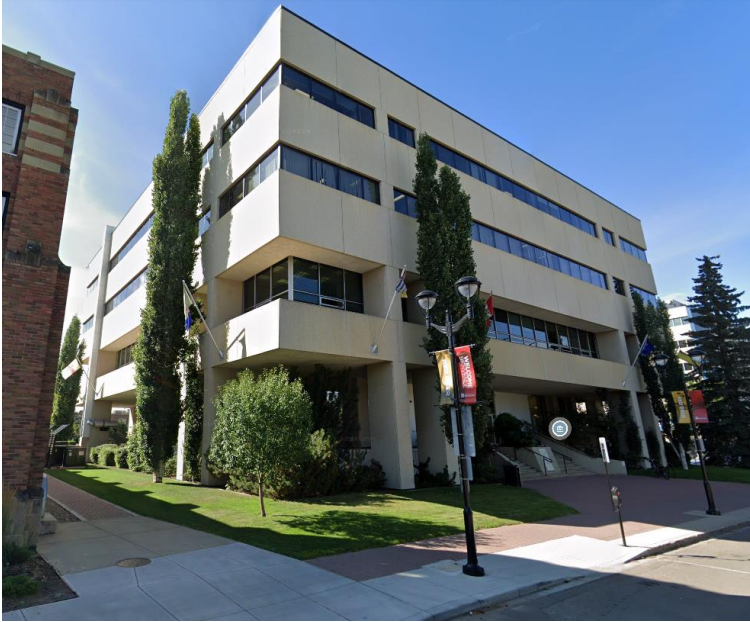
Front and side of building (east and south elevations)
