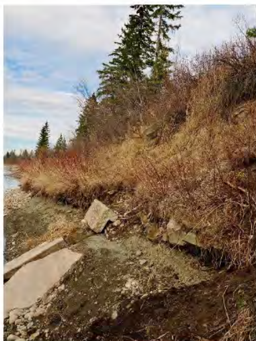
Fig 6: Slump debris immediately downstream of eroding gabion structure.
