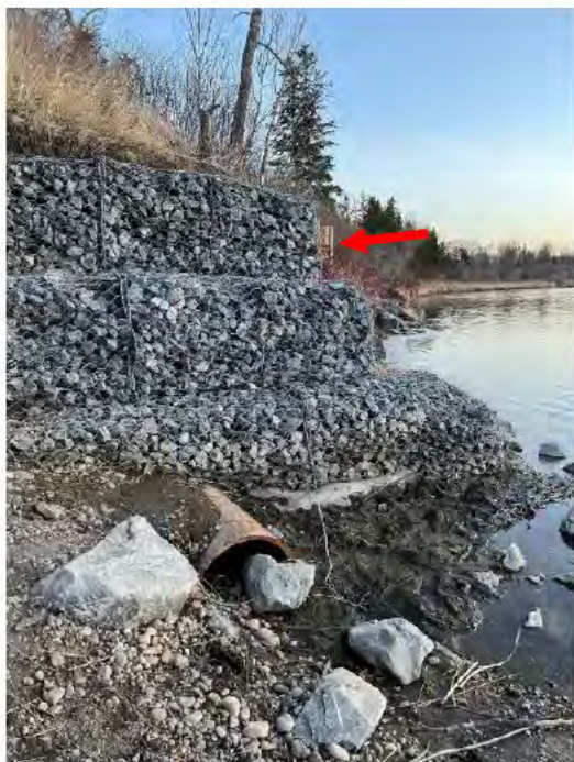
Fig 4: Gabion structure built to stabilize the bank downstream of the old landing site. The red arrow marks the railing above the former landing site.
