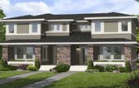
Semi-detached housing without front garage.
