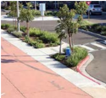
Coloured concrete in median paving area.
