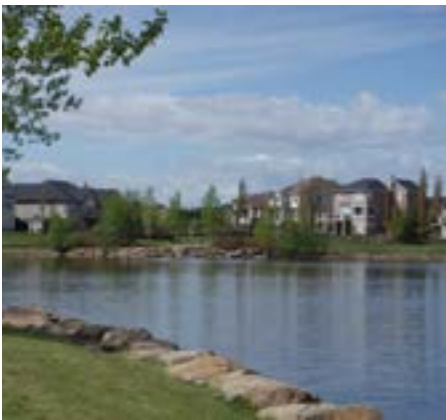
Stormwater management pond.
