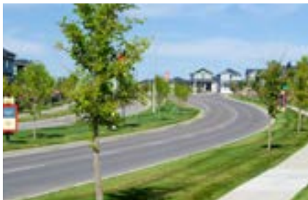
Example of separated sidewalk.
