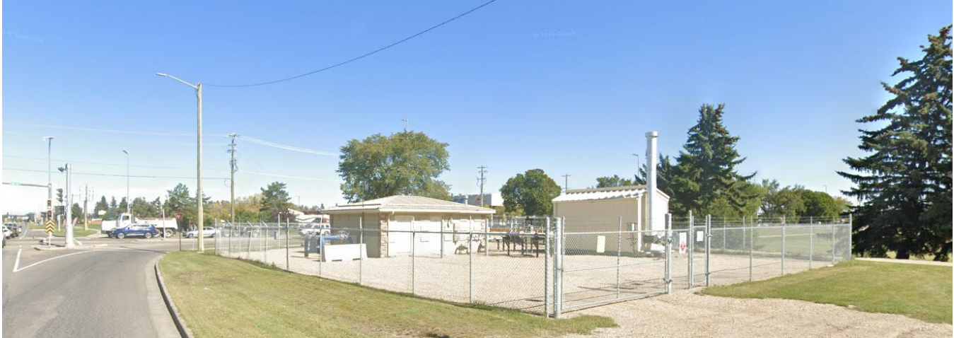
Figure 3: Proximity of Utilities 1
