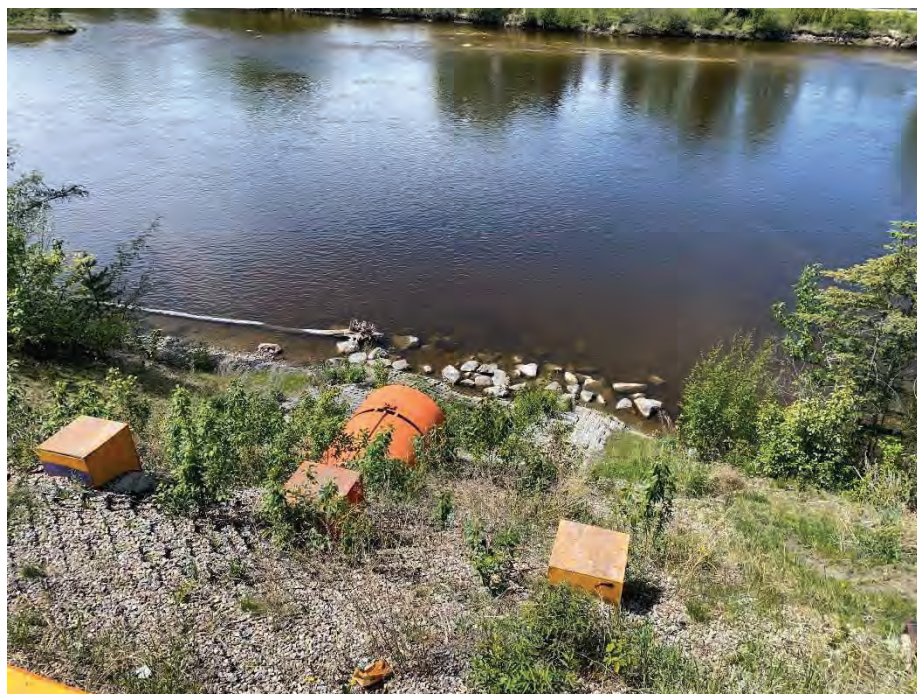
Photo 6: Outfall with the above slope reinforced with geoweb and outlet area protected by articulated concrete blocks at middle of site. Facing north.
