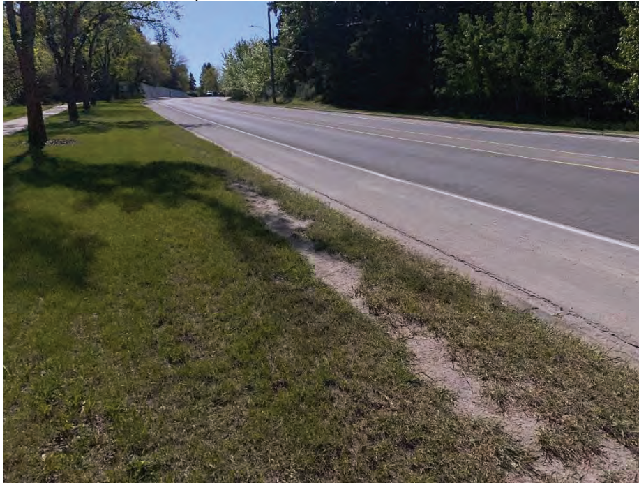
Photo 1: Spruce Drive and boulevard between Spruce Drive and sidewalk. Facing southeast.
