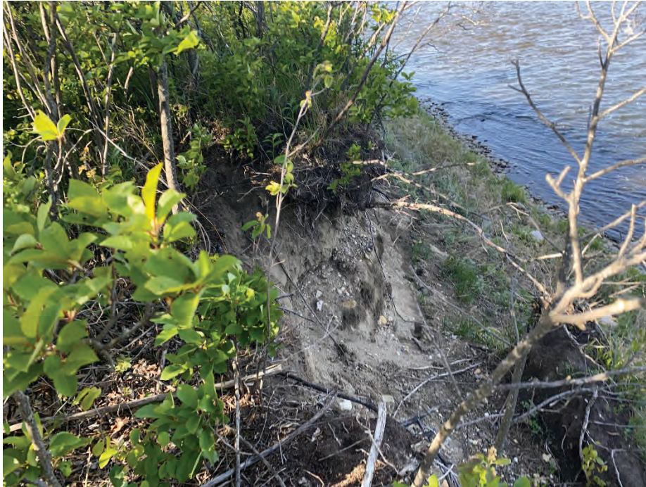
Photo 9: Exposed sandy soil face at failure south of the Kerry Wood entrance. Facing south.
