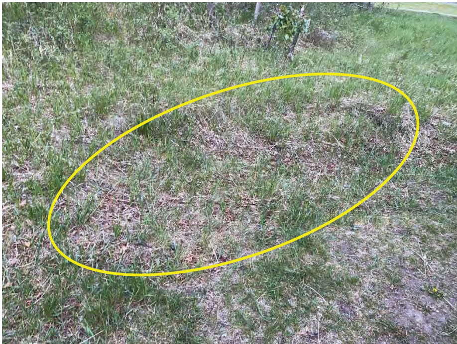
Photo 10: Ground depression between crest and trail at southwest end. Facing east.
