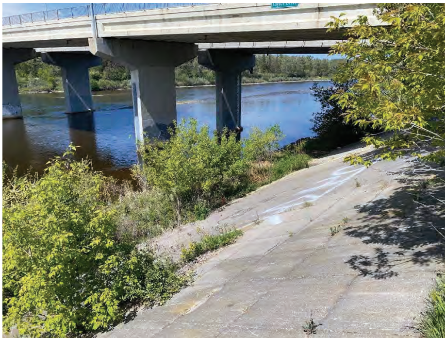
Photo 4: Taylor Drive Bridge and concrete slab armouring on headslope. Looking north.
