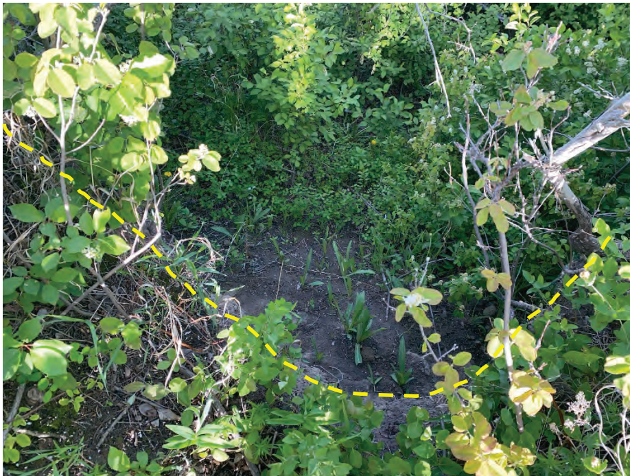
Photo 14: Slide observed on riverbank across from the Community Living Society building. Facing northwest.
