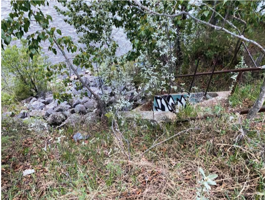
Photo 9: Southwest outfall. Facing north.
