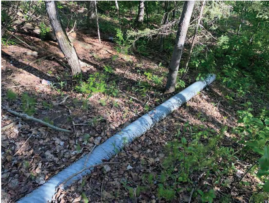
Photo 15: Perforated CSP drain northeast of former Elks building directed downslope. Facing northwest.
