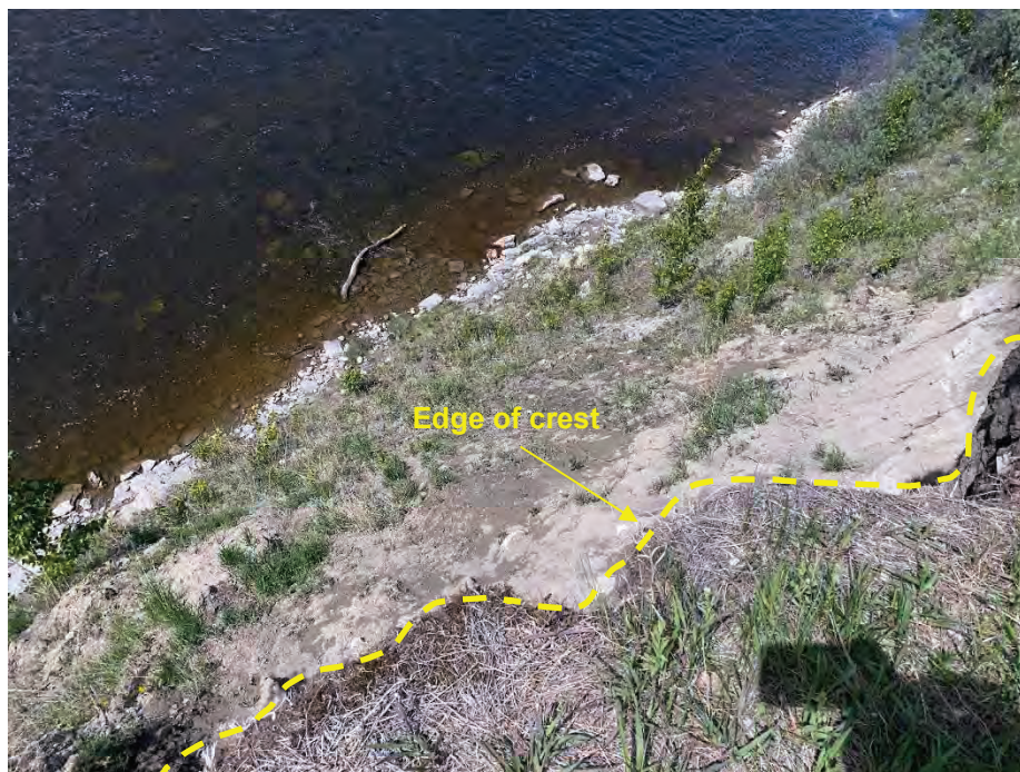
Photo 8: Historical slump at southwest end. Facing down (north).
