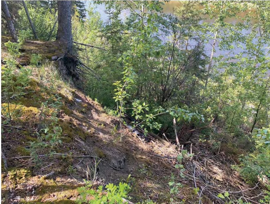
Photo 7: Historical slide behind Lot 15. Facing northwest.
