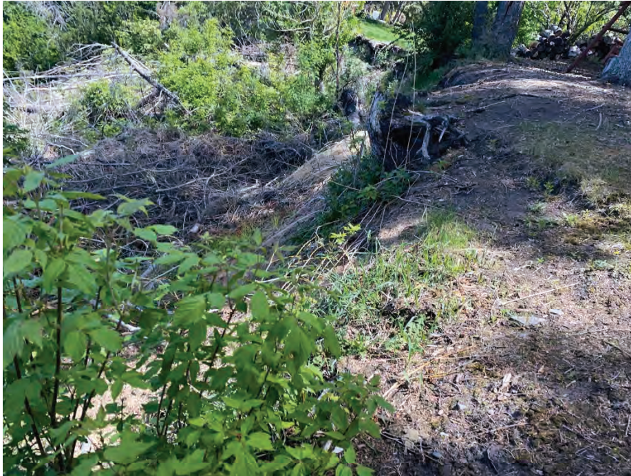
Photo 9: Landslide at Lots 17 and 18, taken from Lot 17. Facing east.
