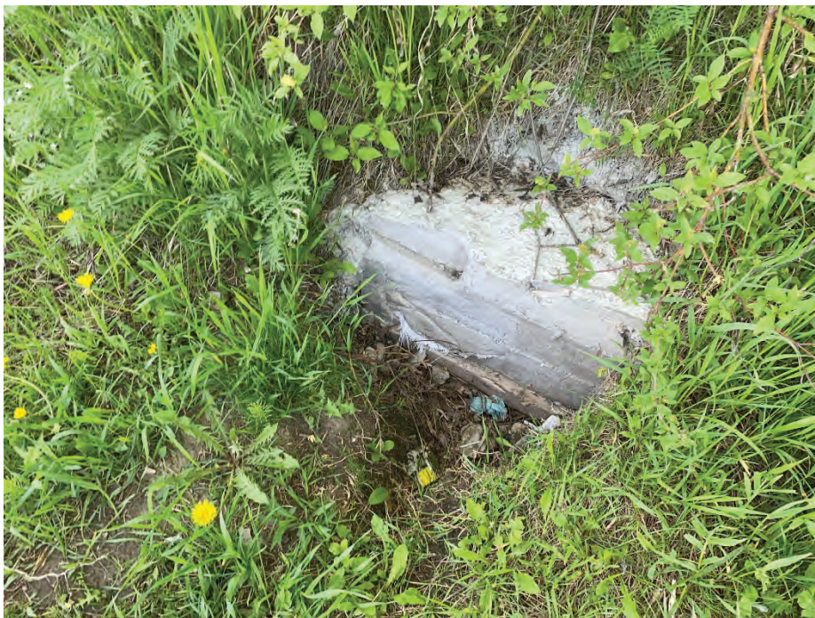
Photo 12: Grouted outfall across from the Parkland School. Facing east.
