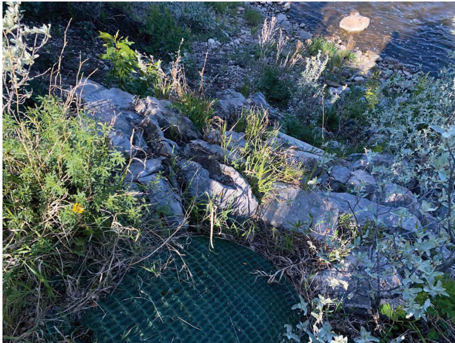
Photo 7: Erosion control blanket and riprap on riverbank slope. Facing southwest.
