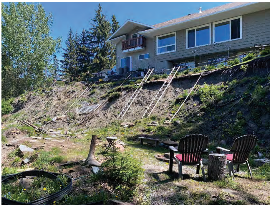
Photo 4: Backyard, landslide backscarp showing ~3.5 m drop. Facing northeast.
