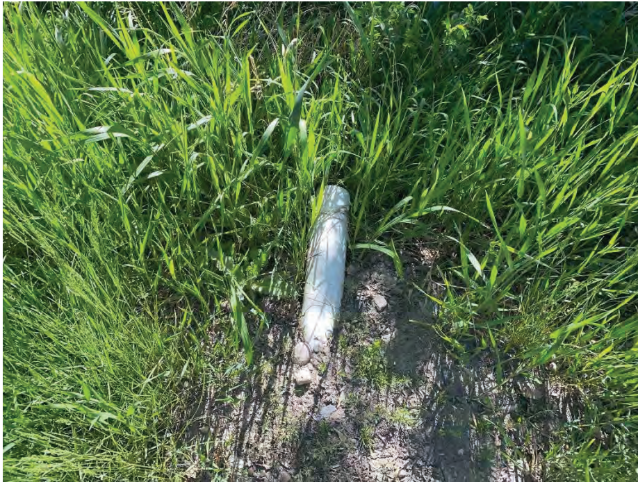
Photo 11: PVC drainage pipe east of former Elks building directing onto slope. Facing east.
