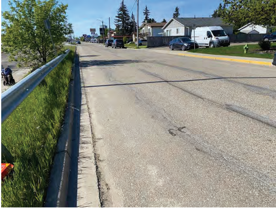
Photo 1: Sealed cracks on Gaetz Ave Service Road. Facing south from mid-section.
