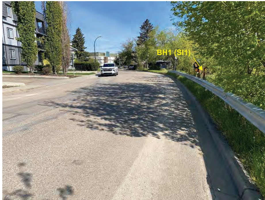
Photo 2: Sealed cracks on Gaetz Ave Service Road. Facing northwest from mid-section.
