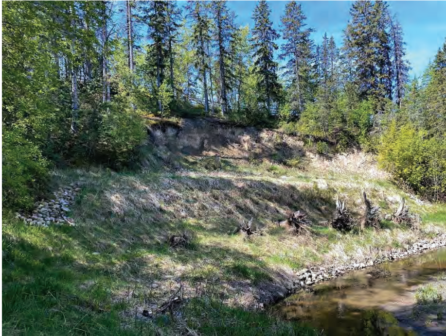
Photo 7: Landslide area on south bank of Waskasoo Creek, note exposed scarp face. Facing southwest.
