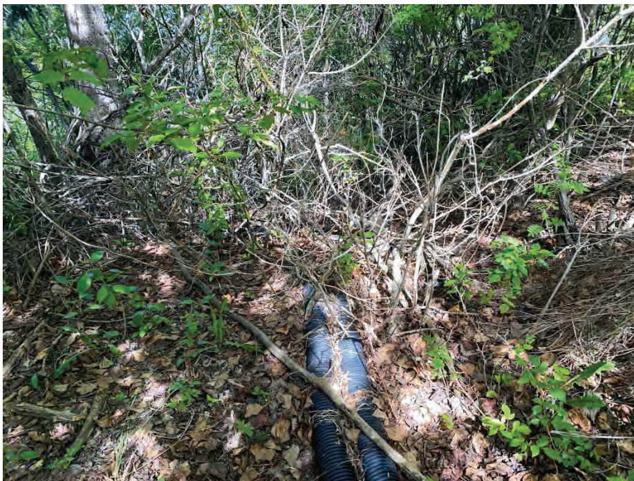
Photo 8: Two pipes behind between Lots 15 and 16 running towards river slope. Facing north.
