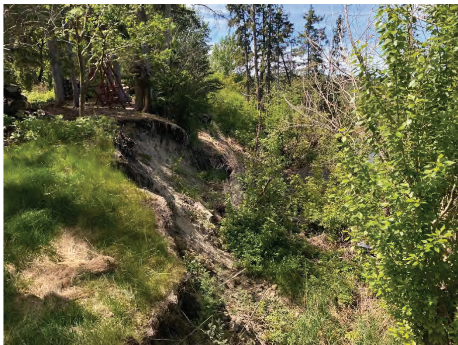
Photo 12: Landslide behind Lot 18, from east extent of slide. Facing west.
