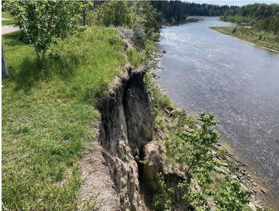
Photo 7: Historical slump at southwest end. Facing west.
