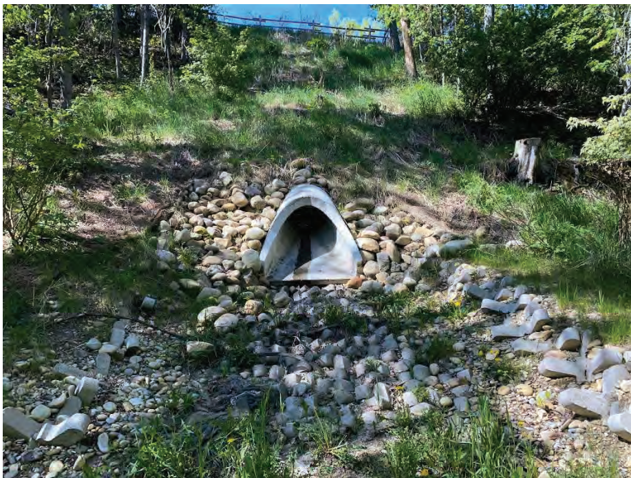
Photo 8: Outfall west of creek. Well vegetated above outfall. Facing southwest.
