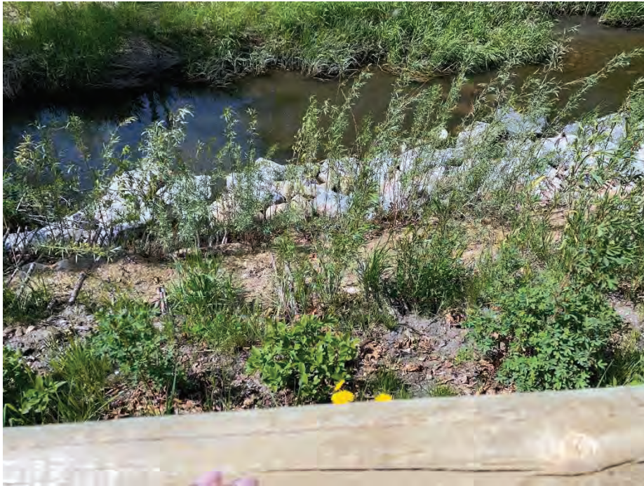
Photo 11: Creek below west slope. Riprap and brush layering on creek edge. Looking west.
