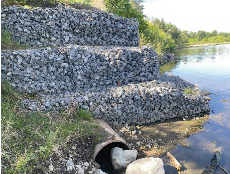
Photo 13: Southern outfall with gabion basket wall. Facing southeast.
