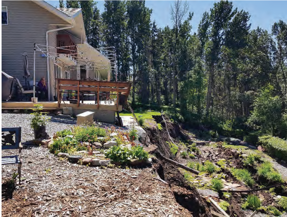
Photo 3: Side yard and deck at crest of slope, facing south.
