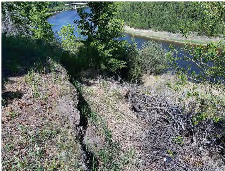
Photo 2: Slide area behind Lot 7. Facing west.
