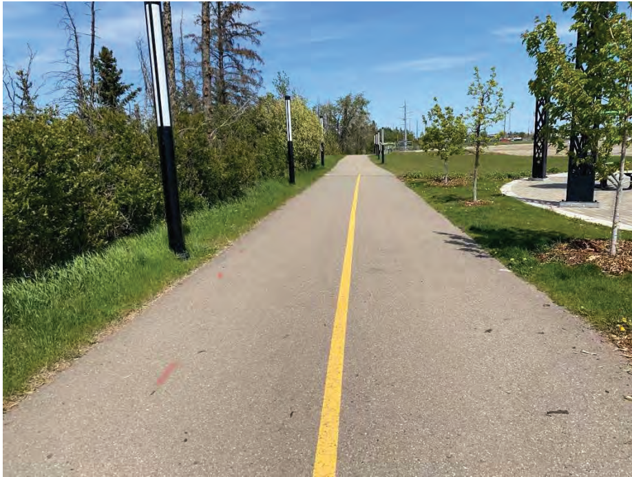
Photo 1: Trail asphalt in good condition. Facing northeast.
