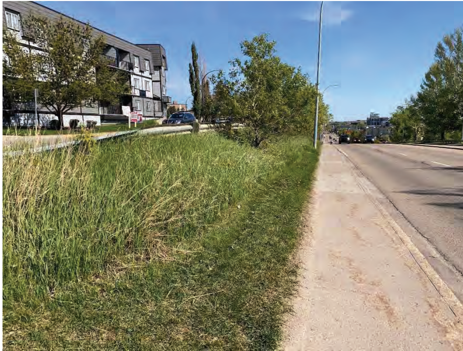
Photo 7: Slope at south end of embankment. Facing north.
