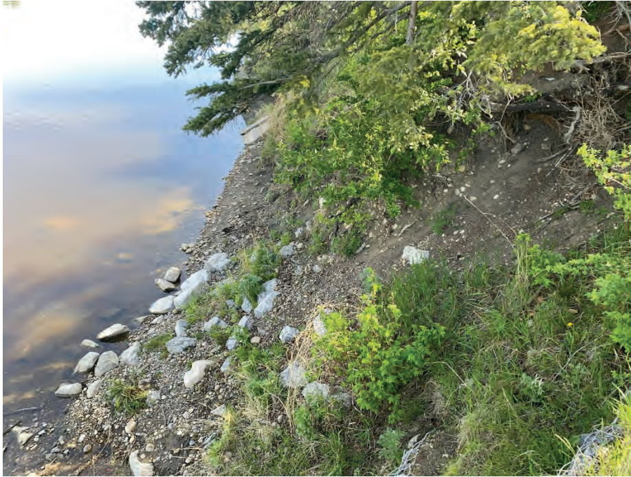
Photo 15: South historical failure area, near 59 Street. Facing northeast.
