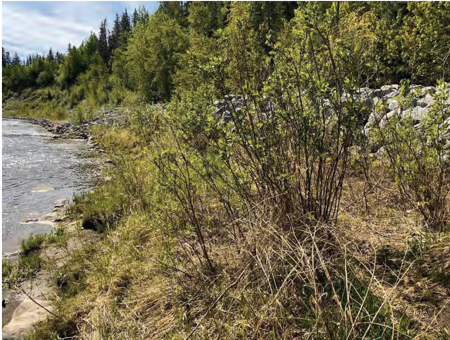
Photo 5: Toe of riverbank with riprap armouring. Looking southwest.
