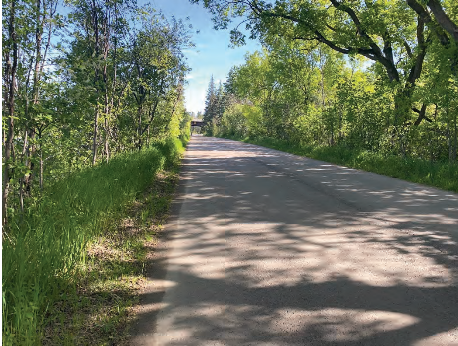
Photo 1: 45 th Avenue asphalt in good condition. Looking north.
