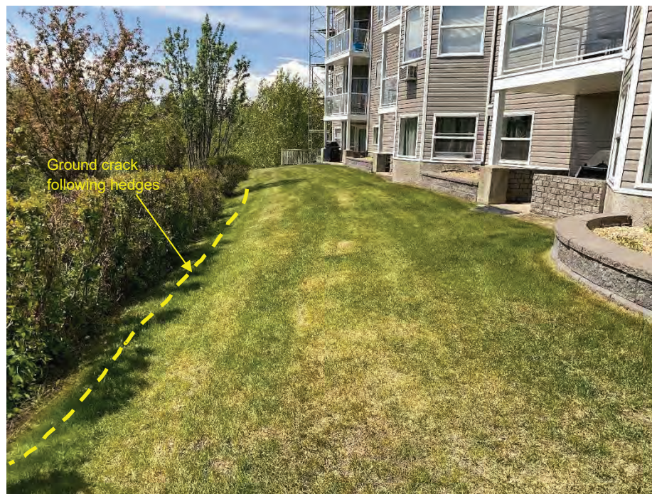
Photo 2: South yard. Looking west.
