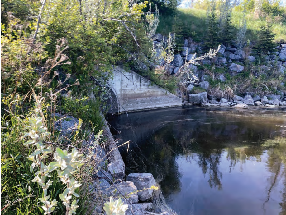
Photo 11: Outfall across from Parkland School. Facing south.
