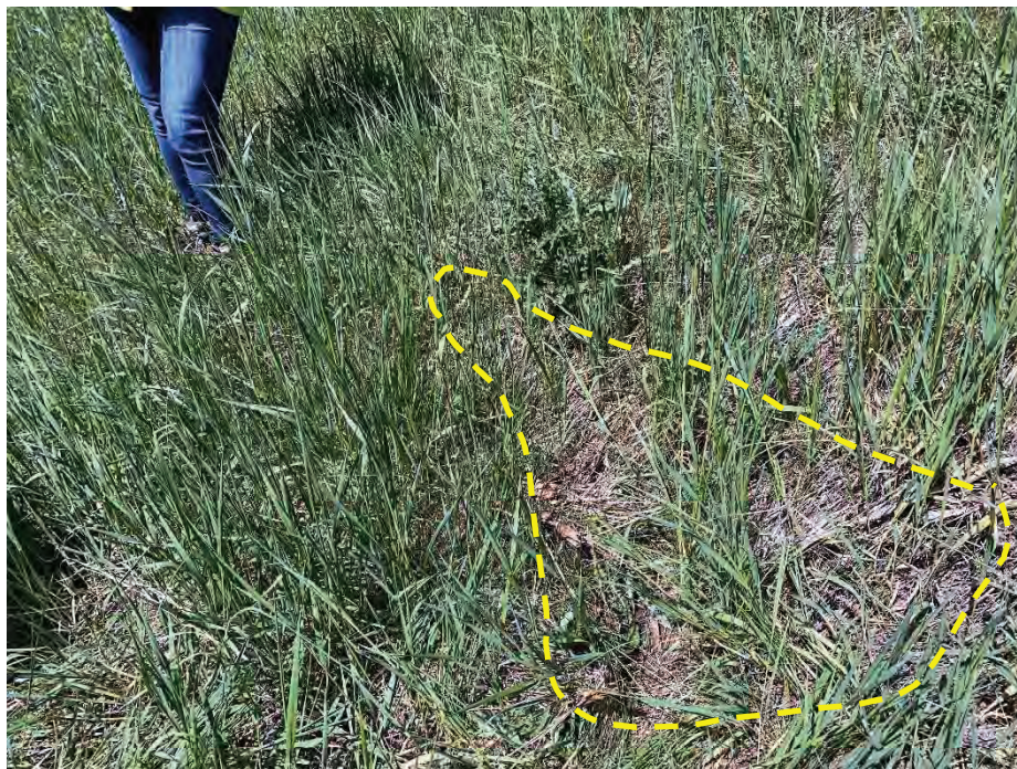
Photo 8: Small depression on south slope face, close to the toe. Looking northwest.
