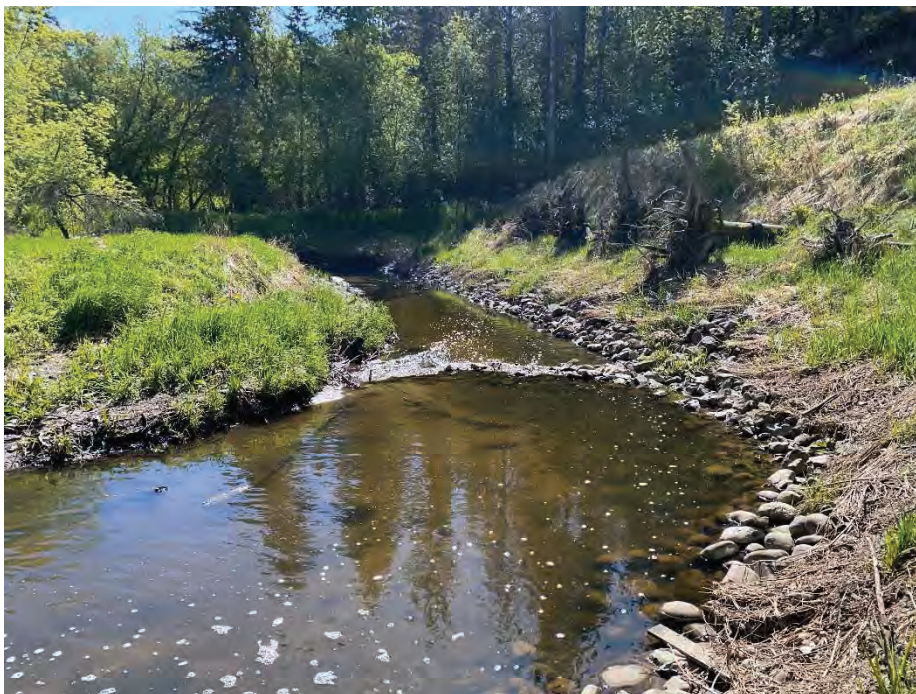
Photo 6: Waskasoo Creek bend with bank armoring. Facing southeast.
