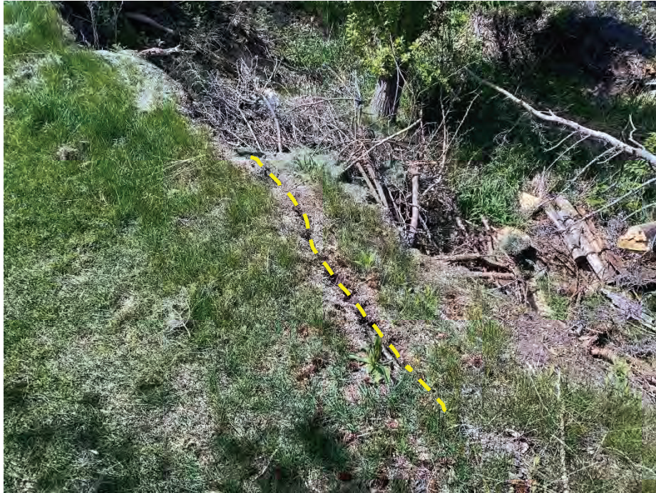
Photo 13: Ground cracking behind Lot 18, looking northwest.
